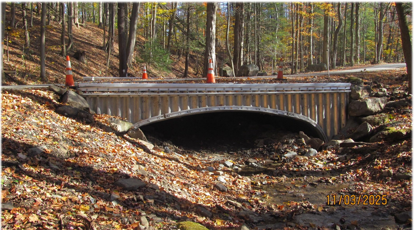
(After): Stream reconnected allowing aquatic organism passage.
