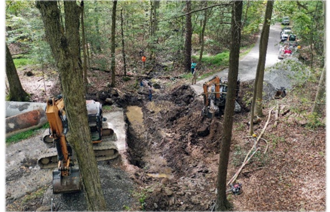
Drone image of roadway being excavated for new structure.
