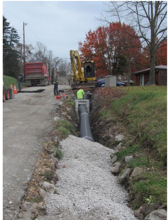
New sewer system being connected to existing drainage system.
