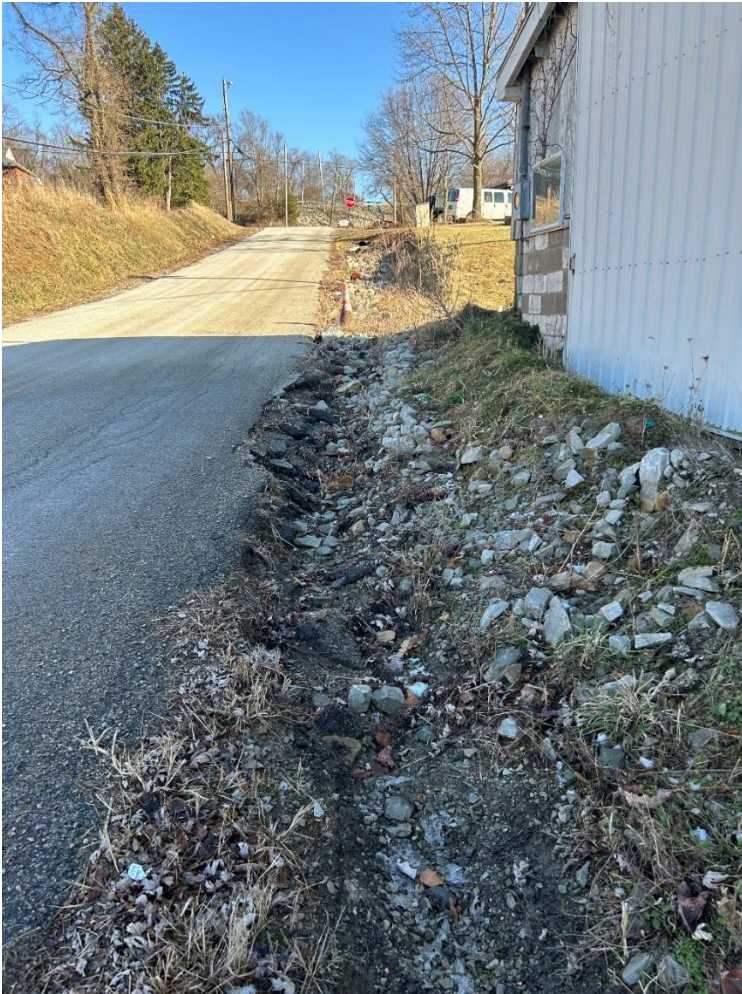
Left: Eroding ditch line from Route 51 drainage.
