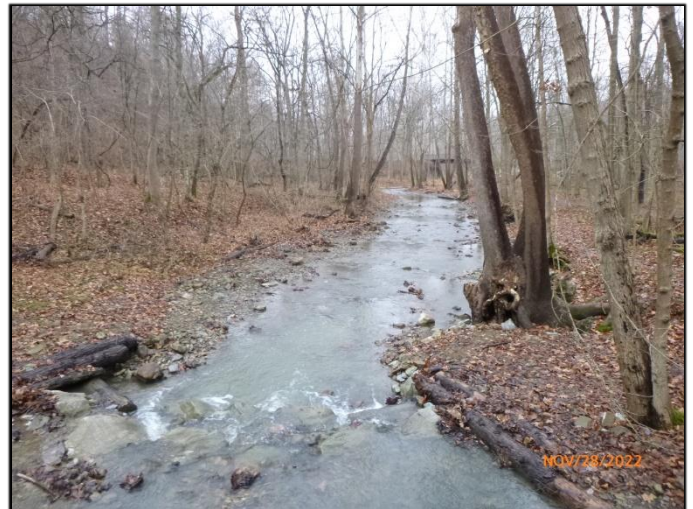
Phase 2A fish habitat structure: log-framed cross vane with rock throat centralizes stream current and stabilizes streambanks.
