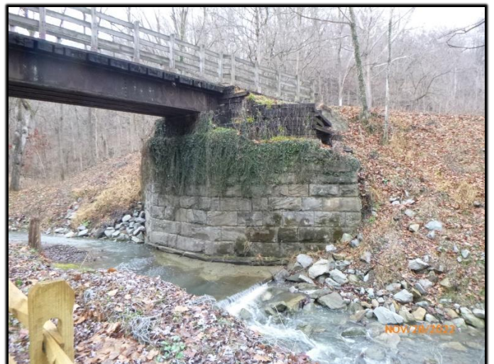
Concrete added stability to bridge foundation to minimize future erosion.
