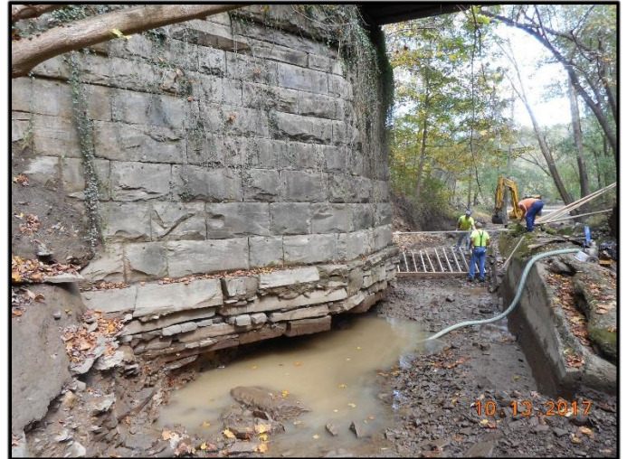
Crews stabilizing the eroded foundation of the bridge.
