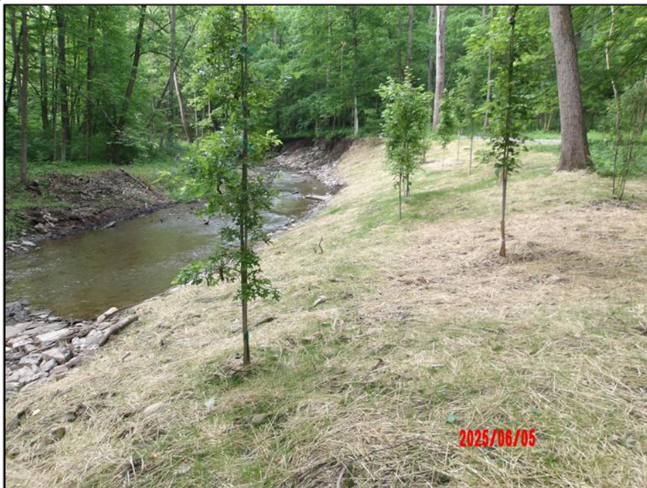
Streambank finished with riparian buffer and grass seed.
