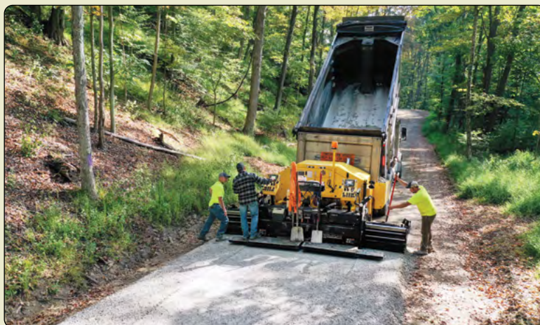
Drone photo of driving surface aggregate (DSA) being installed.
