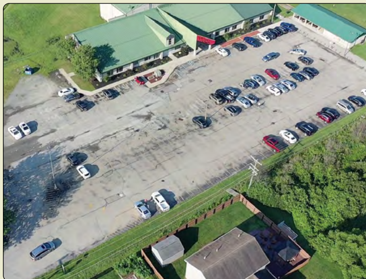
Before: Drone photo pre-construction.
