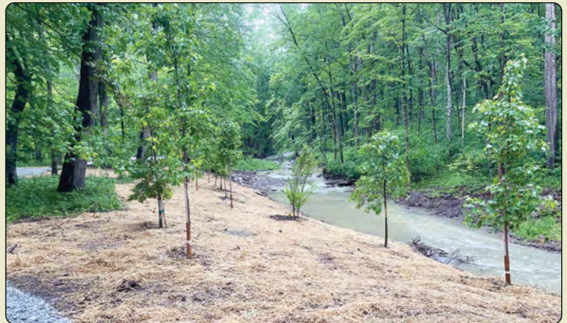
After: Bank grading, single log vane deflectors and native tree plantings were utilized to stabilize the banks.
