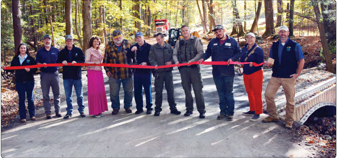
Celebrating the installation of an aluminum box culvert on Sugar Run Road, St. Clair Township, l-r : District Water Resource Specialist Kelly Brestensky; Penn State Center for Dirt and Gravel Road Studies Dave Creamer; Harshman Civil Engineering Group, LLC Rich Rush; State Representative Leslie Rossi; Wayne Mills of Mills Excavating; St. Clair Township Supervisor Dennis Rudnik; PA Fish and Boat Commission SGT. Frank Mehalko and Waterways Conservation Officer Matt Kauffman; Brandon Mills of Mills Excavating; State Senator Joe Pittman's Field Representative Gina Jones; District Manager/CEO Rob Cronauer.
