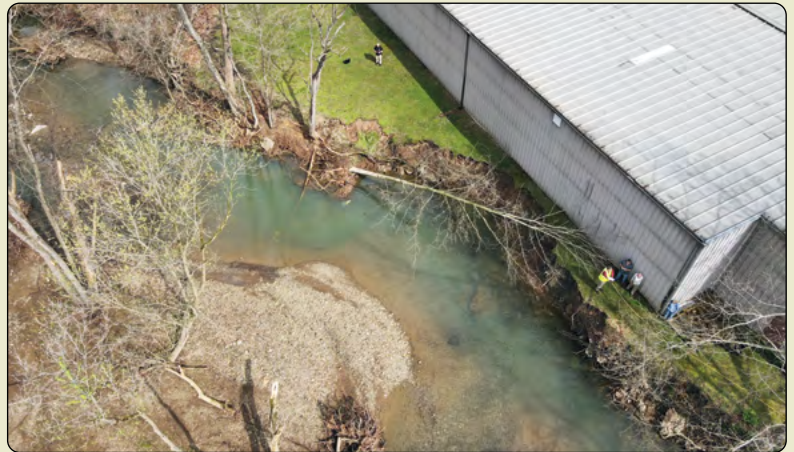
Before: Aerial view showing the proximity of the erosion.
