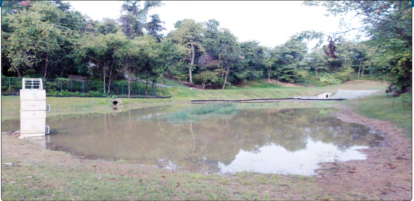
This Norwin School District stormwater basin was retrofitted with a new forebay inflow and outlet riser for more efficient stormwater and erosion/sediment control. In this photo, the freshly planted grass around the basin will help stabilize its banks.
