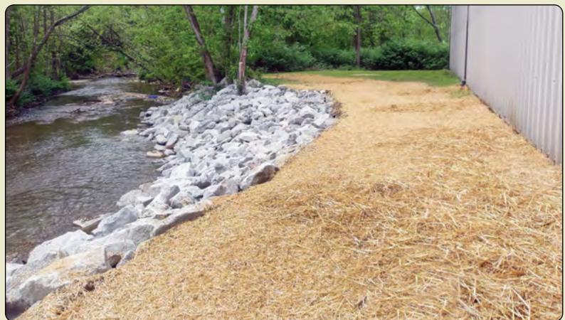
After: Stabilized streambank and yard area restored.
