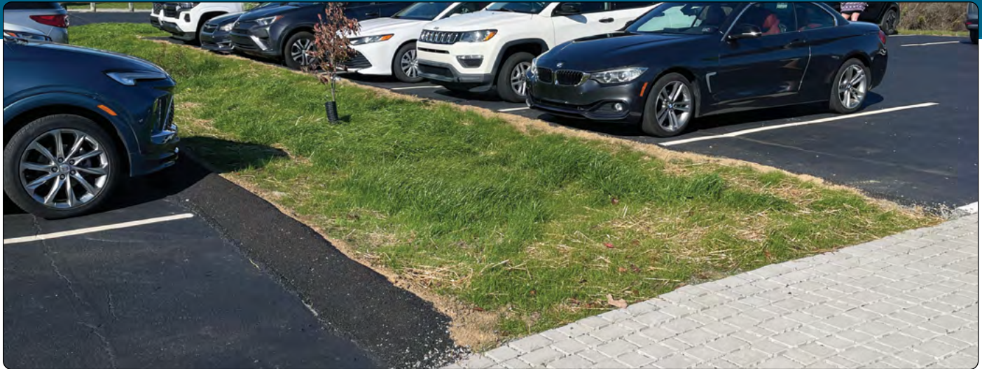
Landscape islands installed in the parking lot at the Regional Family YMCA of Laurel Highlands allow stormwater to infiltrate into the ground, rather than run off. Pedestrian walkways made of permeable pavers also allow stormwater infiltration (see pages 14-15).
