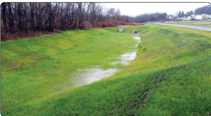
Here's a post construction view of the stormwater management bioretention basin at Derry Business Park. An amended soil mix was used for the basin bottom comprising of leaf compost, top soil, and sand. Trees and shrubs are expected to be planted.
