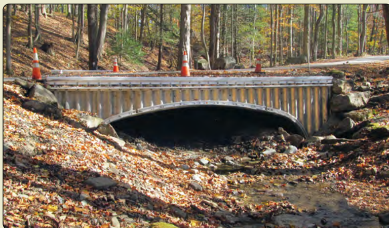
After: Stream reconnected allowing aquatic organism passage.
