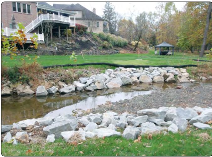
Location of the sanitary sewer line crossing Haymakers Run where stream stabilization took place after the line was installed. Here 55 linear feet of the sewer line were encased in concrete.
