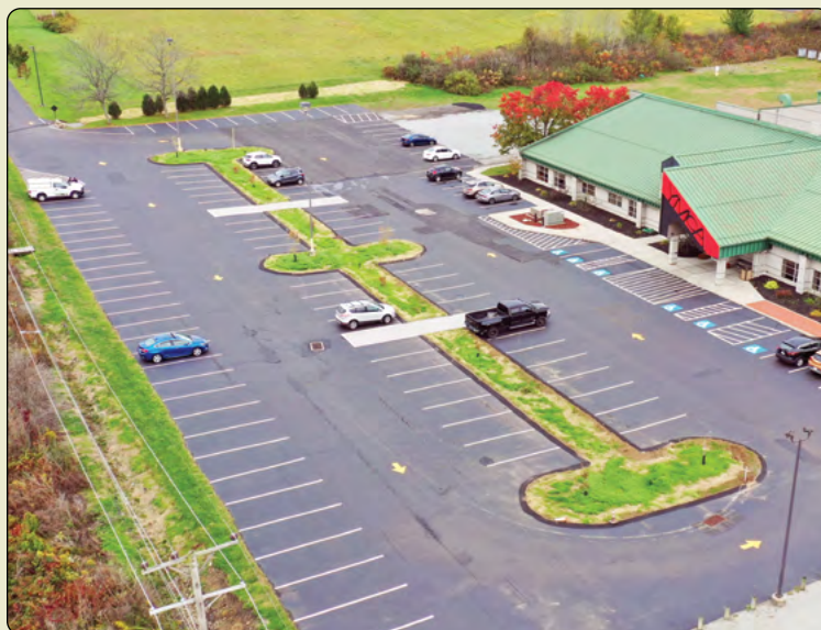
After: Drone photo post-construction.
