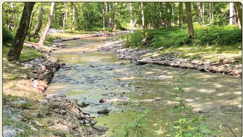
After: Several in-stream fish habitat structures were installed including the log-framed cross vane pictured here.
