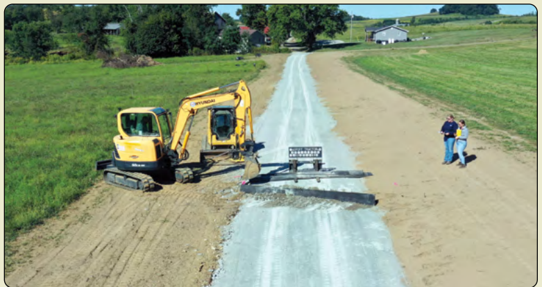
During Construction: Stabilizing the animal walkway and installing conveyor belt diversions.
