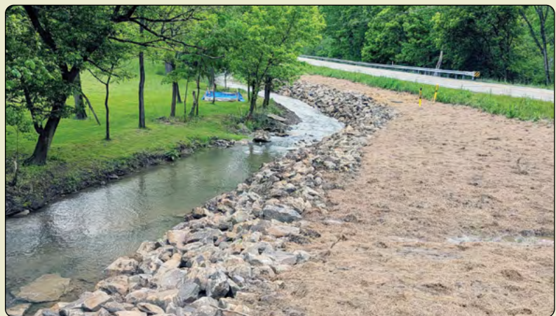
After: Stabilized streambank and yard area restored.
