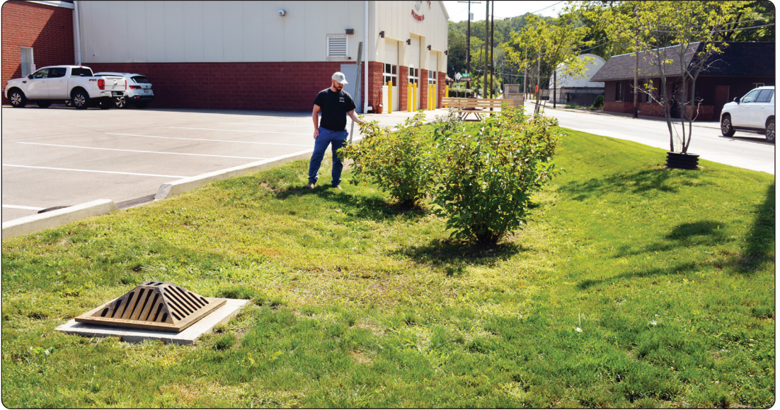
Westmoreland Conservation District Stormwater Program Technician Hank Bradish inspects shrubs growing in a rain garden at the Manor Borough building.
