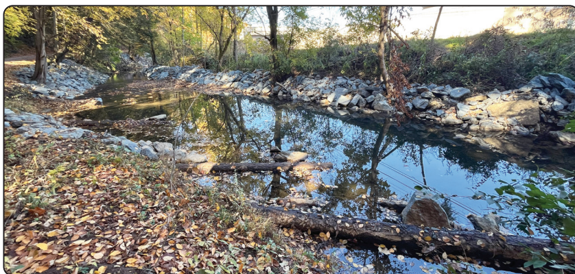
Stabilized streambanks along Turtle Creek in Duff Park, Murrysville
