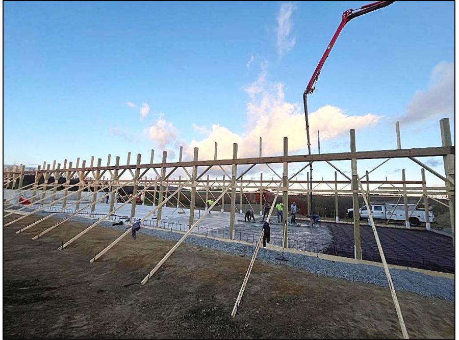
A concrete floor is being poured in a new roofed animal heavy use area with a manure stacking pad.
