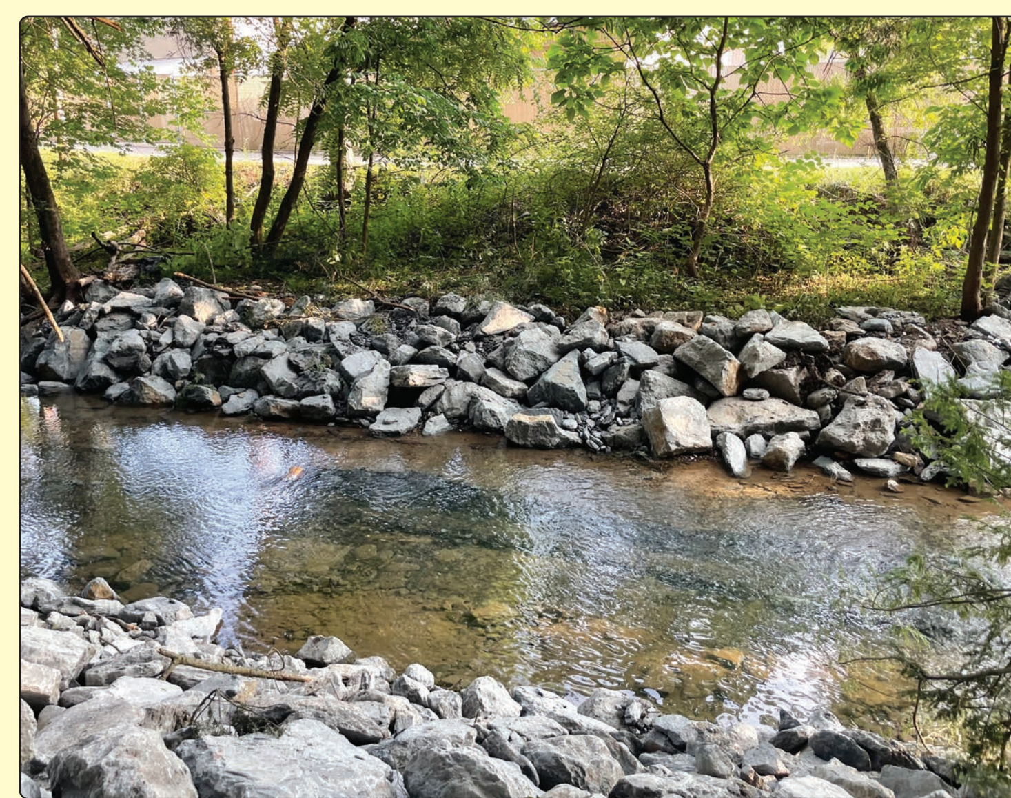
Streambank stabilization along Turtle Creek in Murrsville's Duff Park.
